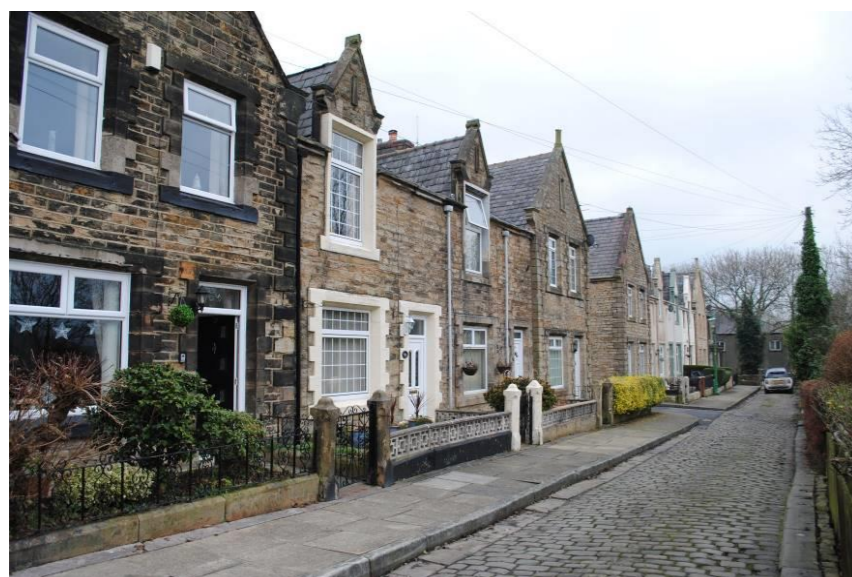
Figure 51 Shuttleworth Street looking east
