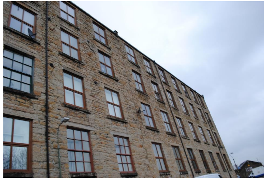
Figure 49 Victoria Mill on Ightenhill Street
