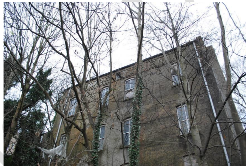
Figure 37 Globe Cinema from Fairmore Medical Practice car park
