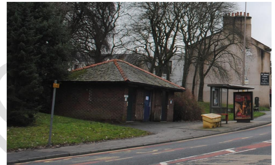
Figure 67 Bus shelter and public toilets adjacent to area of soft landscaping
