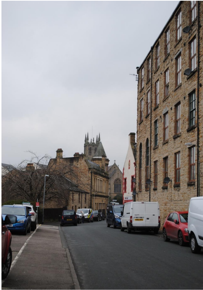
Figure 48 St Leonard's Church Tower from Ightenhill Street
