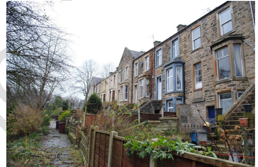
Figure 54 Properties to the west of Shuttleworth Street; rear of Albert Street.
