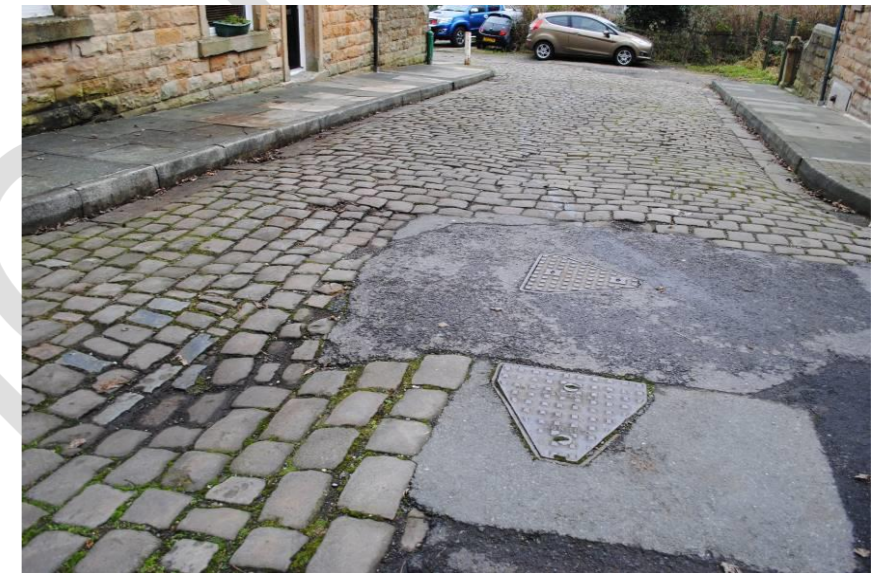
Figure 58 Poor quality surface repair on the corner of Dragon Street and Albert Street.
