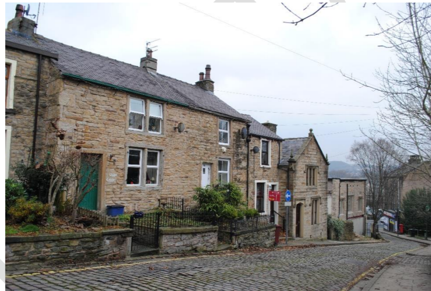
Figure 13 Example of buildings responding to the distinctive sloping.
