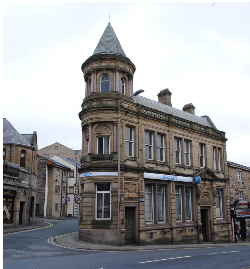
Figure 20 Barclays Bank on Burnley Road
