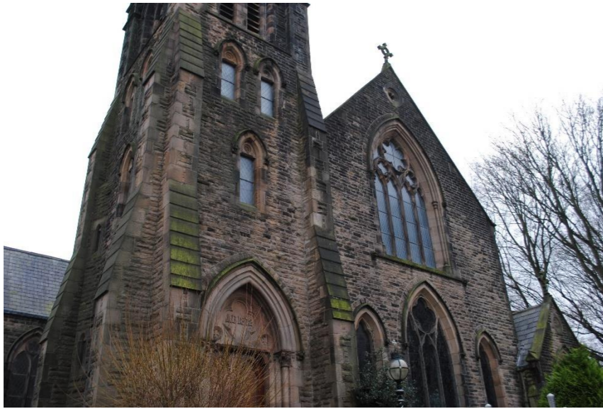
Figure 76 Unitarian Chapel from Church Street
