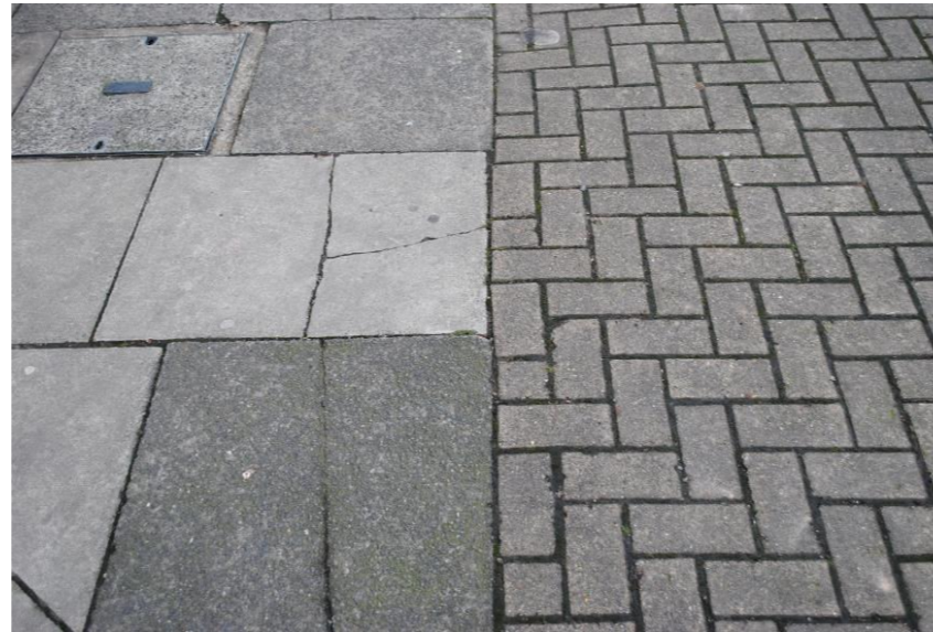
Figure 24 Flagged and bricked street surfaces on the corner of Church Street
